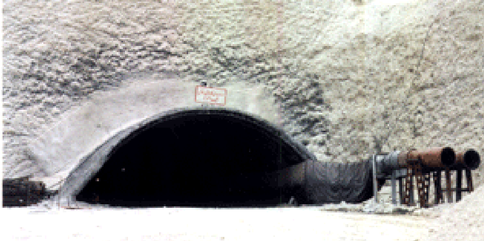
Figure 4: Left tunnel exit (top heading excavation stage)..
